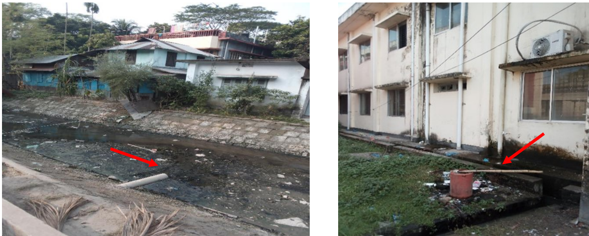
Figure 6: Containment technologies and their connections in Barguna Left: Toilet pit open to a nearby water body, Right: Toilet pipe connected to open environment (Source: Feasibility study 2020-21/DPHE).
