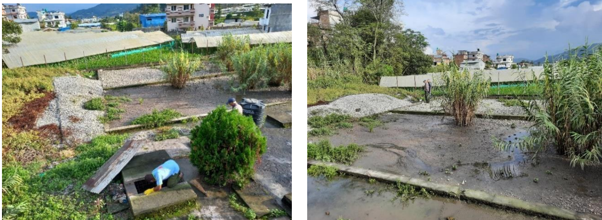
Figure 6: Overview of Nala wastewater treatment plant and overflow constructed wetland.
