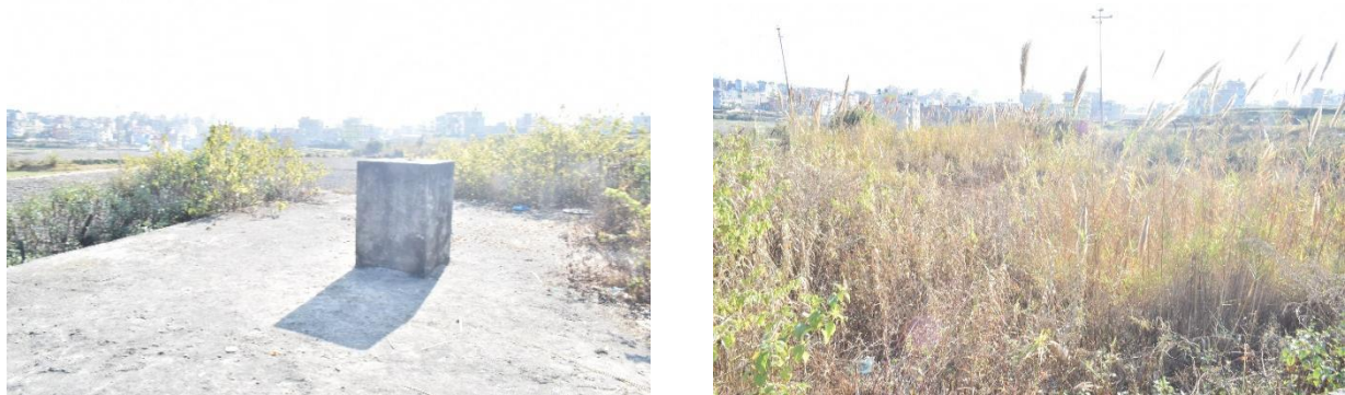
Figure 4: A deserted settler, untrimmed and overgrown reeds in the constructed wetland in Chandeshwori WWTP.
