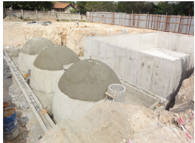
Biogas domes & ABR during construction
