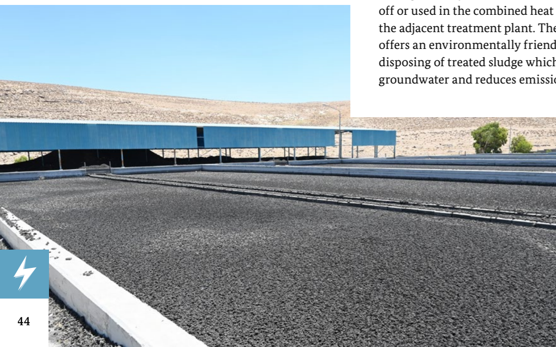
← Sludge management at the Mu'tah Mazar wastewater treatment plant
