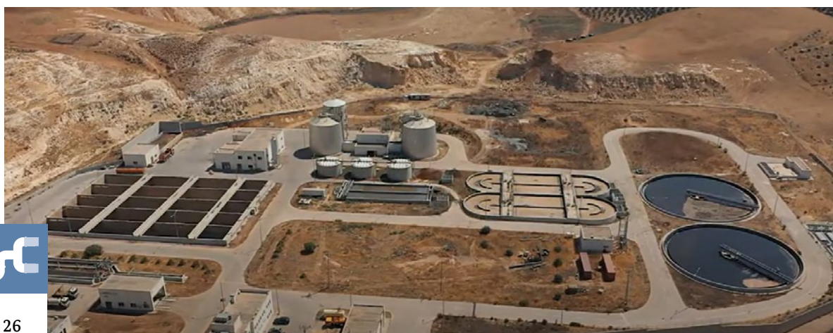
↳ The Wadi Shallalah wastewater treatment plant, in Irbid Governorate (top and bottom)
