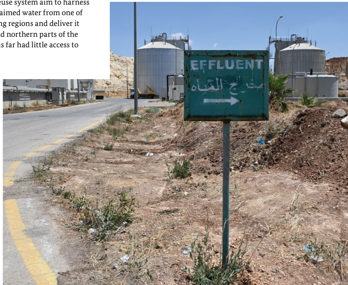
↓ Wadi Shallalah wastewater treatment plant
