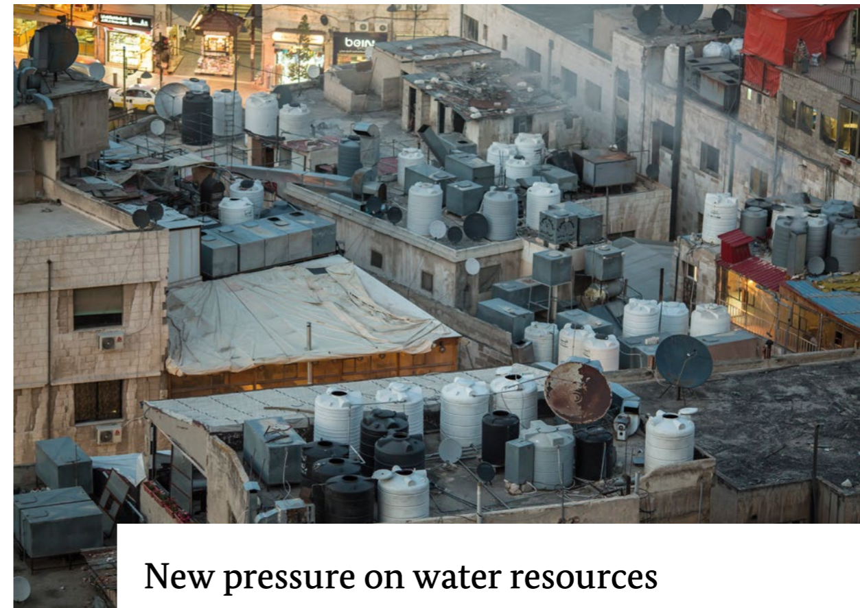
← Water storage tanks on Jordanian rooftops
