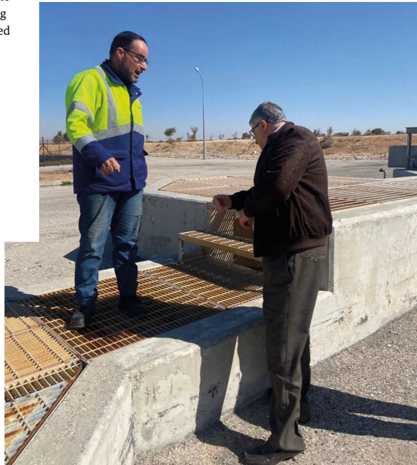
↓ Inspection of a wastewater treatment plant by the Utility Performance Monitoring Unit
