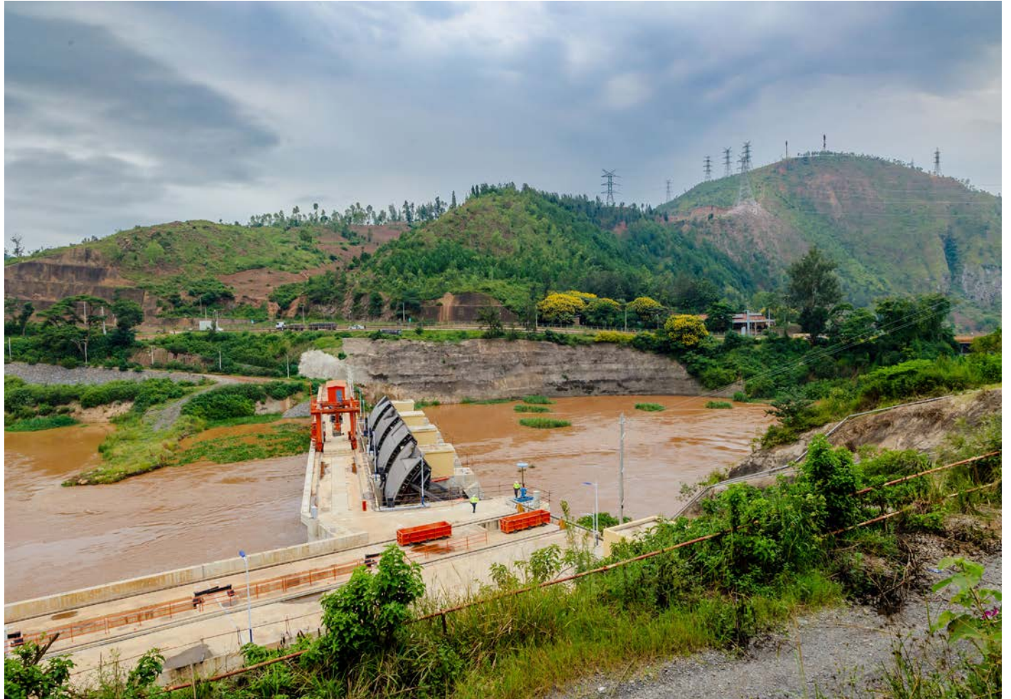
Photo of the Regional Rusumo Hydroelectric Project during the Nile Basin Initiative's Experiential Learning Tour.
