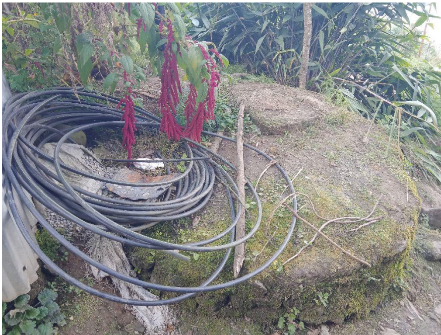
Figure 5: Unlined Pit installed in the household at Phidim Municipality.
