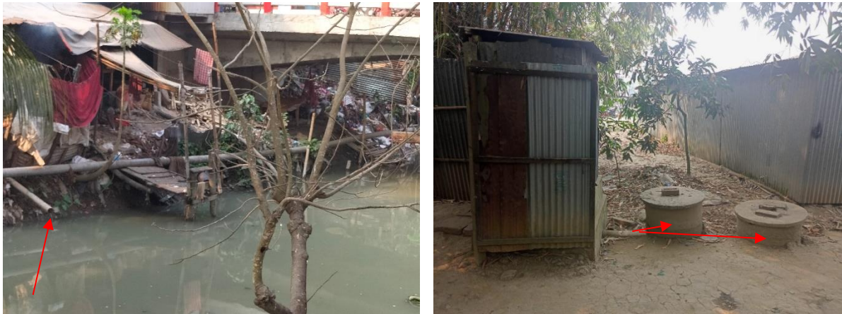
Figure 6: Containment technologies and their connections in Bauphal Municipality. Left: Toilet outlet connected to water body, Right: Toilet outlets direct connected to dual pits. (Source: Field Survey 2023/ O.CREEDS_ WaterAid Bangladesh).
