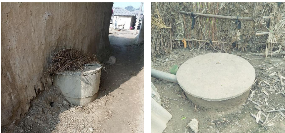
Figure 7: Single pits found in the Kolhabi Municipality.
