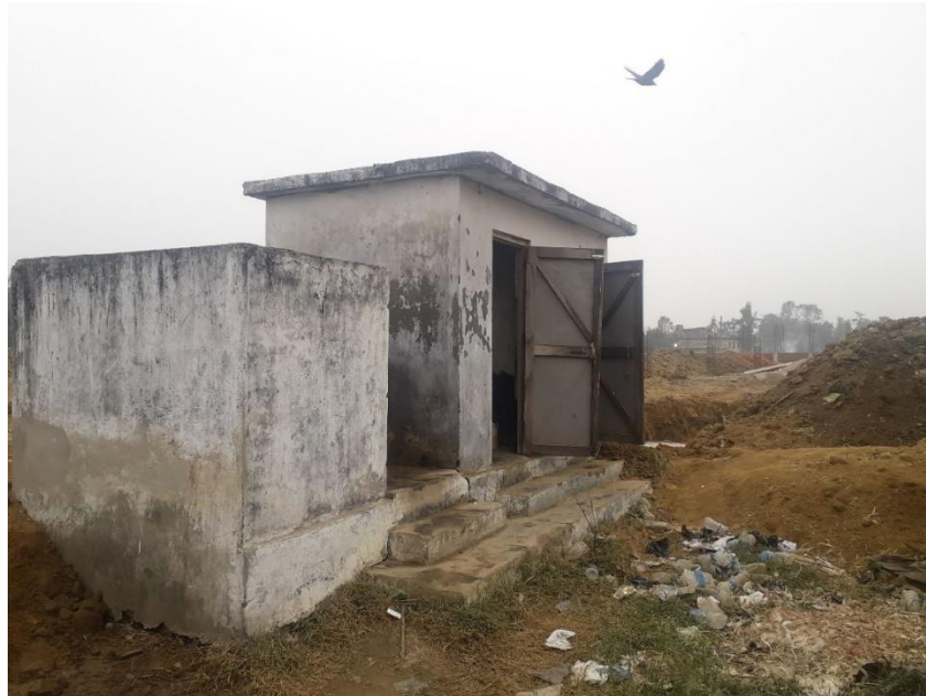
Figure 11: Structure of public toilet located at local marketplace of ward no. 2.
