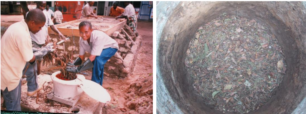
Adding semi composted palm leaves to the base of a Fossa alterna pit in Mombasa, Kenya (left). Two sacks full of leaves at the base of a concrete lined pit in Maputaland, South Africa.
