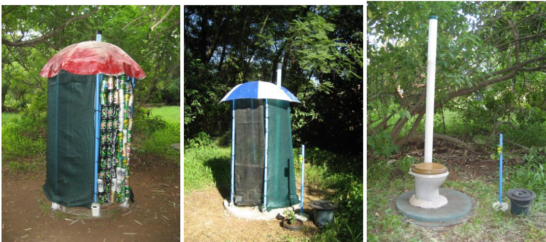
Three of the several demo ventilated Arborloos recently built in my garden. The central photo is a smaller toilet designed for children. The right photo one designed for my “Urban Forest Garden,” filled with trees which provide privacy. Note the simple hand washers – an essential partner to any toilet.
