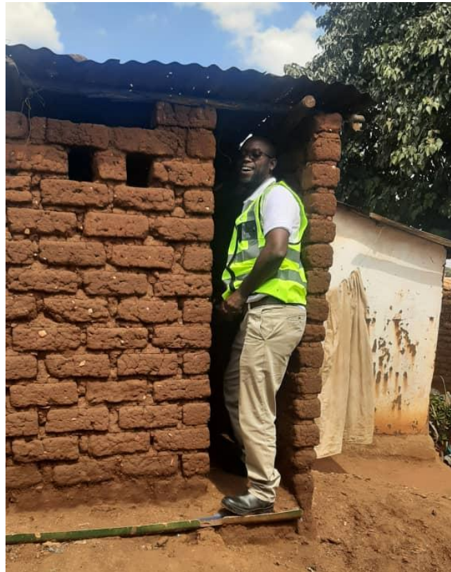
Figure 4: A Pit latrine without slab or lining (Mkwezalamba and Kabika, 2023).
