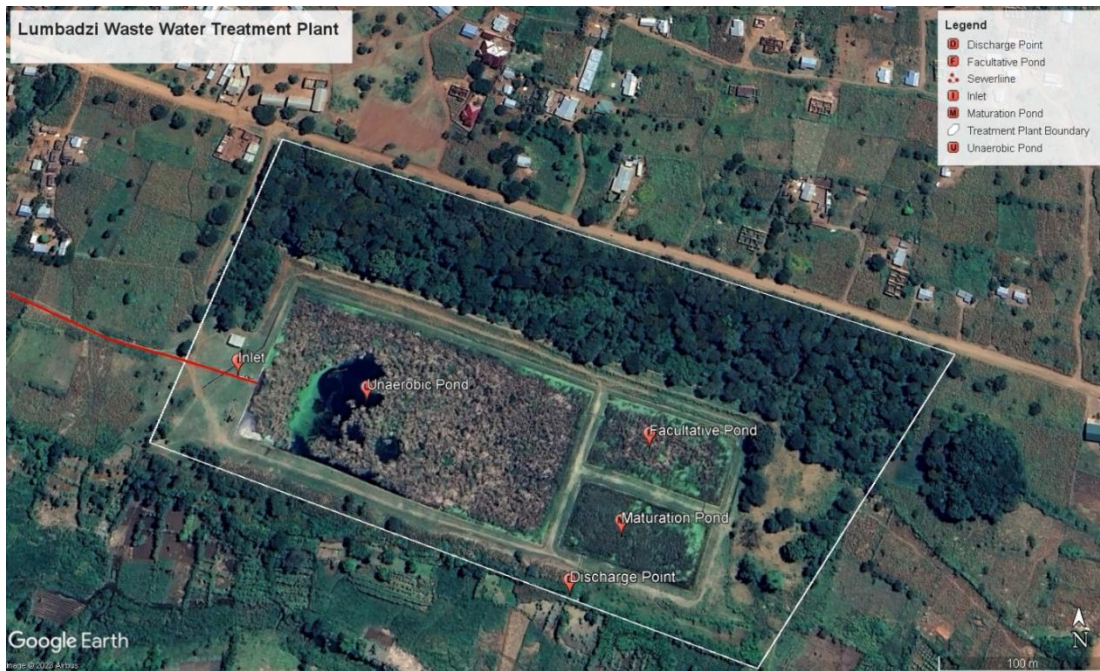
Figure 16: Lumbadzi Wastewater Treatment Plant (Google earth, 2023).
