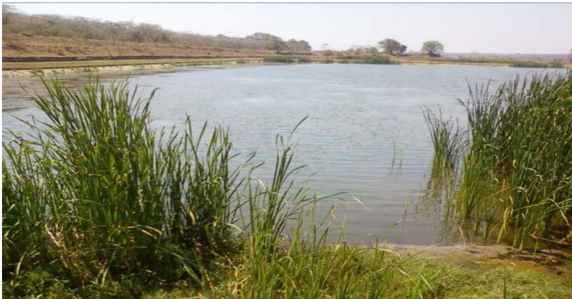
Figure 15: Lumbadzi Wastewater Treatment Plant (Mkwezalamba and Kabika, 2023).
