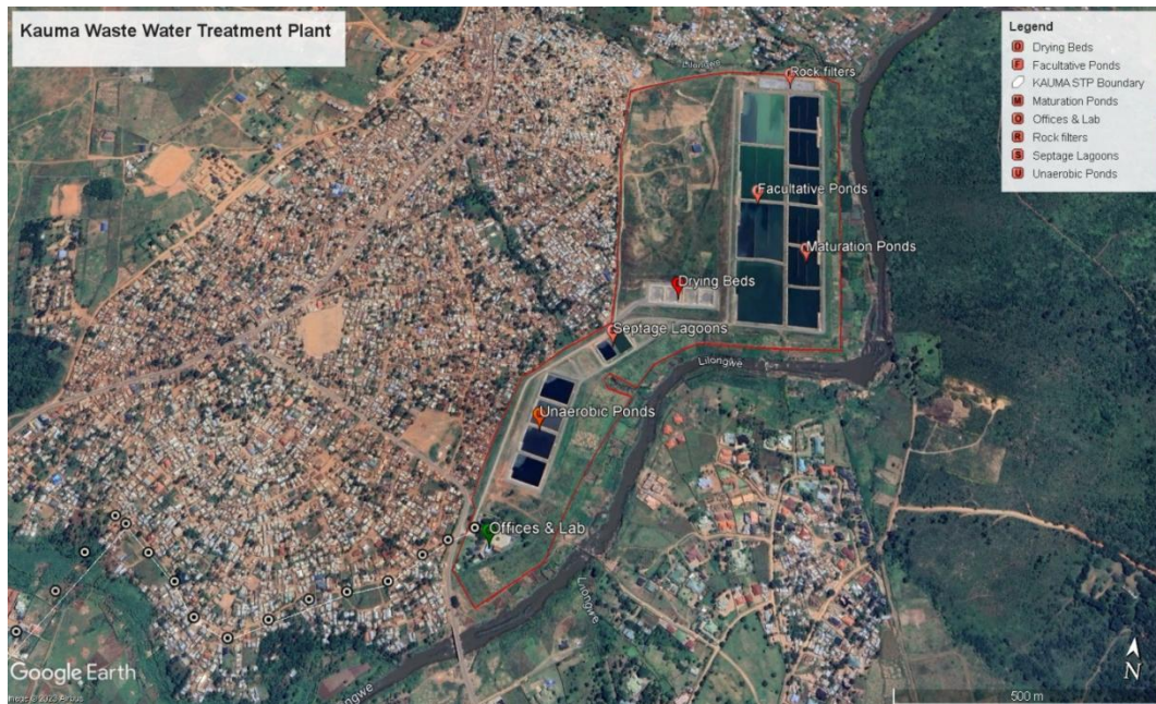
Figure 12: Lilongwe Wastewater Treatment Plant (Google earth, 2023).
