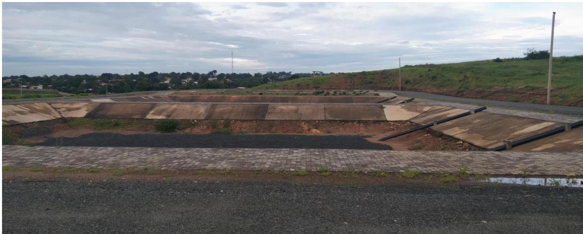
Figure 11: Lilongwe Wastewater Treatment Plant-FS Drying Beds (Mkwezalamba and Kabika, 2023).
