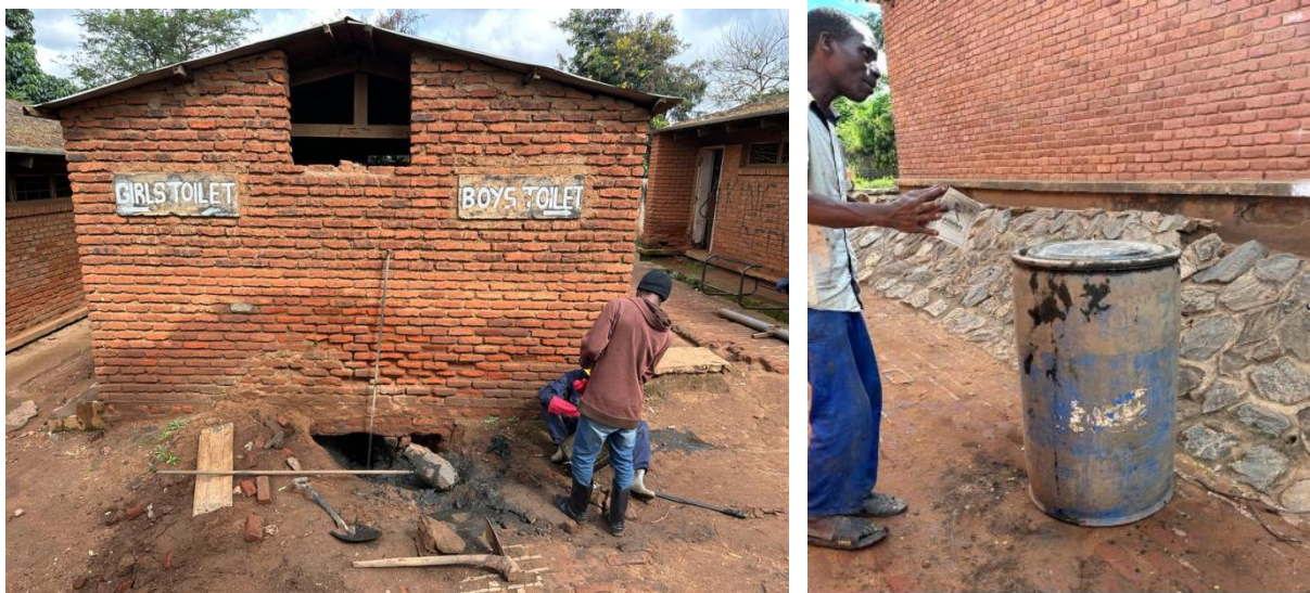
Figure 5: Faecal sludge operators emptying a public sanitation facility (School Toilet) (Mkwezalamba and Kabika, 2023).
