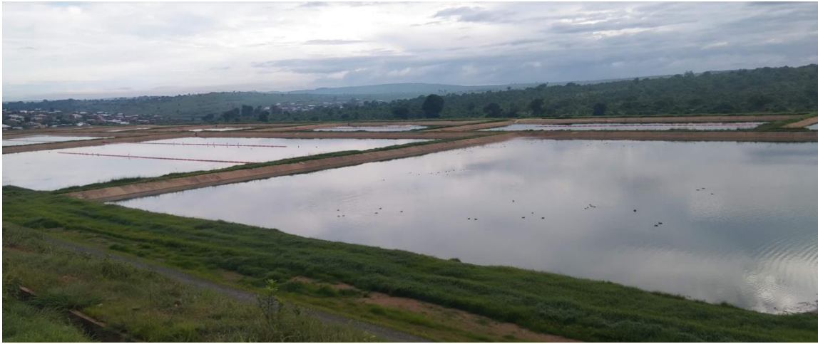
Figure 10: Lilongwe Wastewater Treatment Plant-Facultative & Maturation Ponds (Mkwezalamba and Kabika, 2023).
