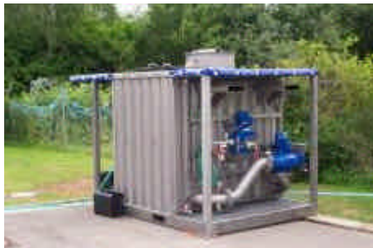
Figure 8: Membrane container installation
