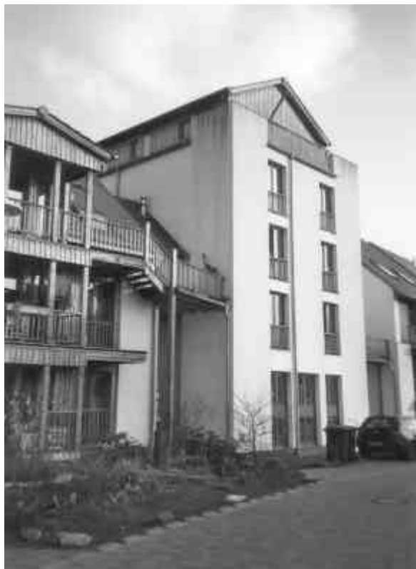
Figure 1: Four story building with public Kindergarten
