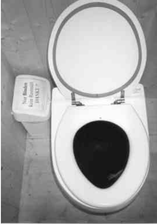
Figure 4: Toilet stool with black removable insert and sealing
