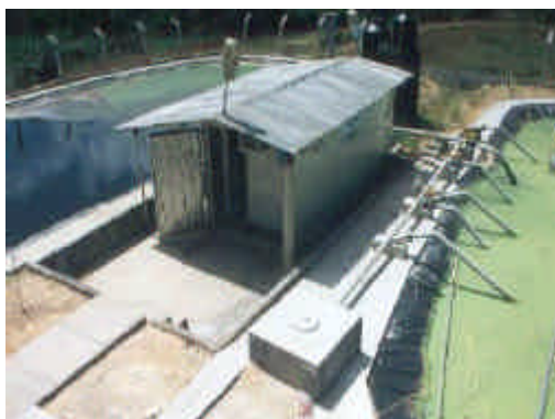
Figure 7: TBW-InWaSia-System for water, nutrients, energy production, recycling and reuse from industrial waste water in Cuba.
