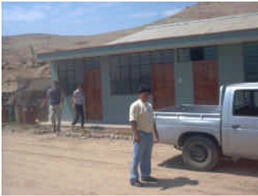
Figure 15: Anaerob-aerob waste separation, treatment and recycling plant in Canete, Peru.
