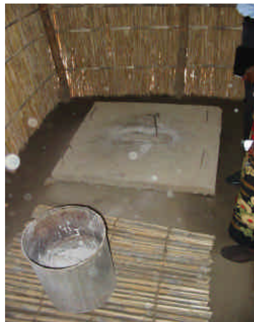
Figure 3: Fossa alterna , a shallow reinforced pit, soil-composting toilet in use in Mozambique (Source: Water Aid)
