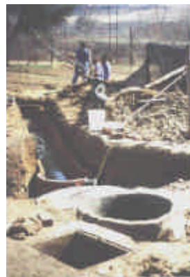
Figure 2: Canal and treatment for distribution of nutrients and treated waste water, Lesotho.
