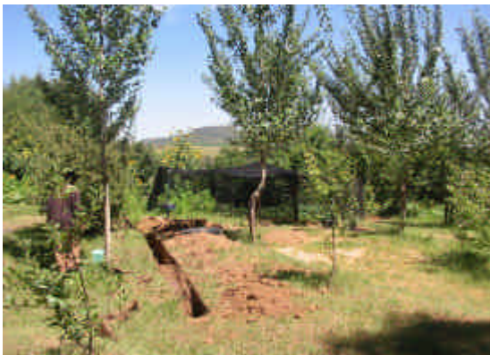
Figure 7: Construction work in Lesotho
