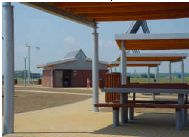
Figure 7: view from the pergolas to the solar toilet
