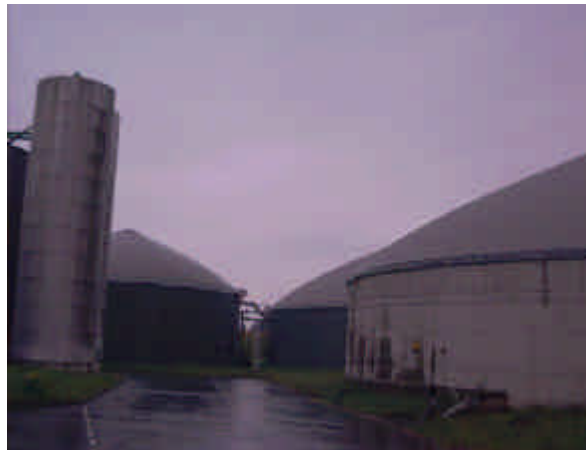
Figure 12: Digesters; treatment plant for municipal, agricultural and industrial wastes.
