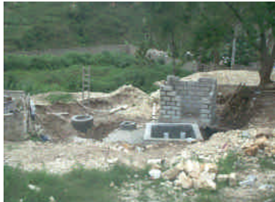
Figure 14: Integrated waste treatment and fertilizer distribution plant, use of toilet and green biomass energy, Thomassin, Haiti.
