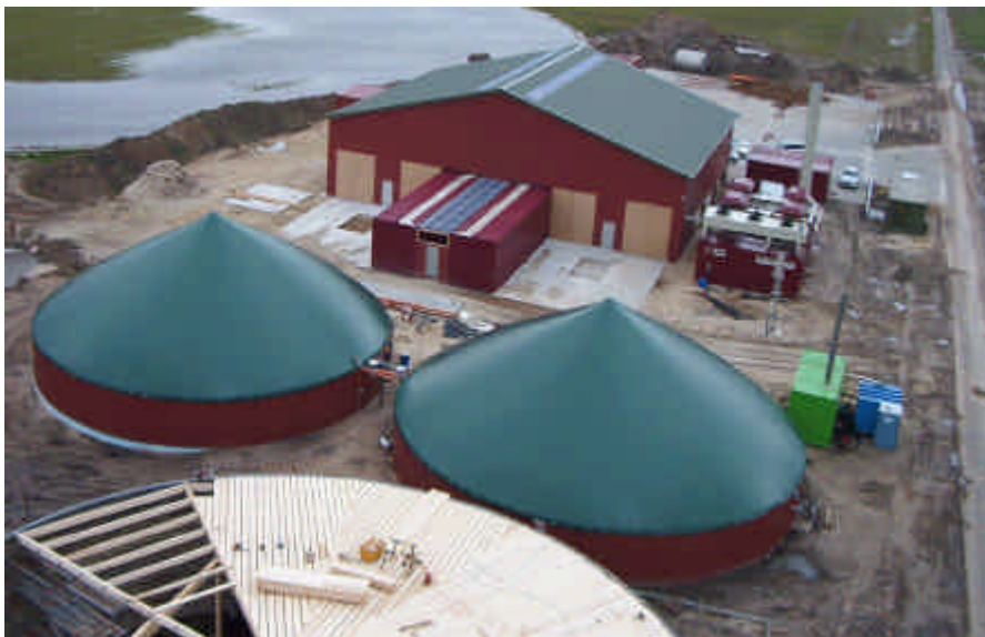
Figure 2: Aerial view of a wet-dry combination biogas - plant
