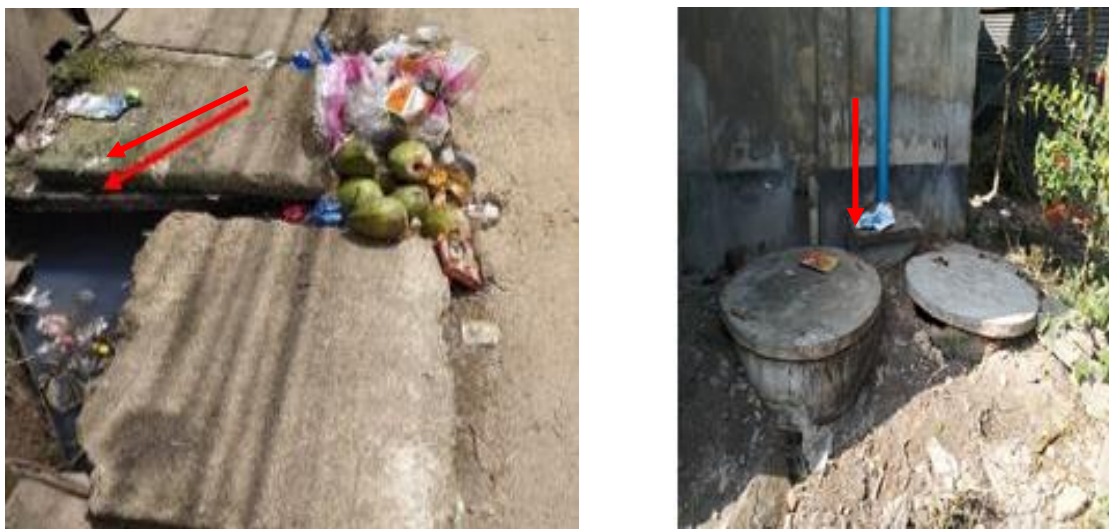
Figure 6: Containment technologies and their connections in Rajshahi. Right: Toilet Pit Connected to open drain, left: Toilet pipe connected to open environment. (Source: Feasibility study 2020-21/DPHE ).
