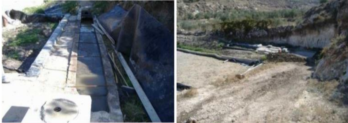
Figure 5: WWTP of Nuba.
