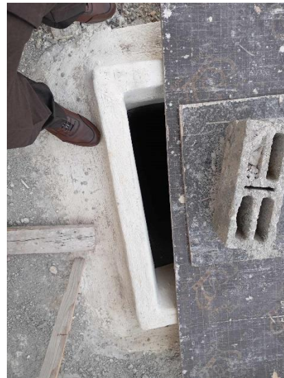
Figure 7: Septic tank en Cesspit zonder outlet.
