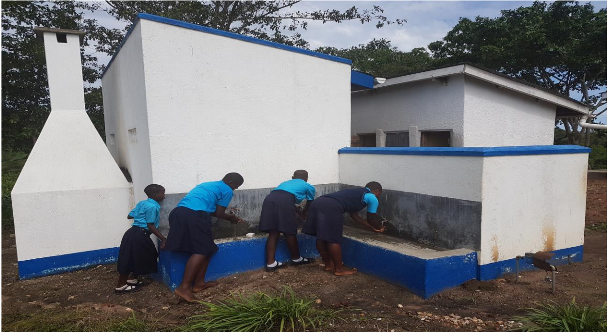
Photo a school toilet with an incinerator built close to the girls' changing room to promote privacy and dignity
