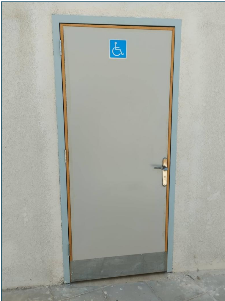
Figure 6: Door of constructed toilet for PWD (source internal from S4M in Jordan in 2022)
