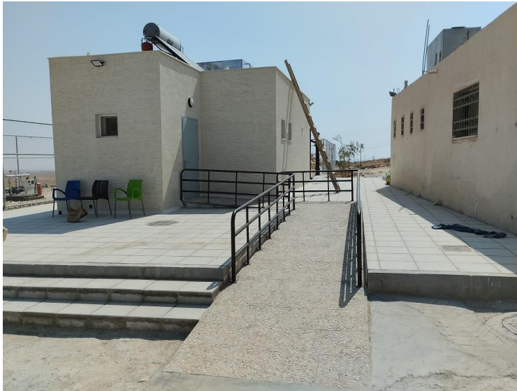
Figure 4&5: Ramp with appropriate surface and slope (source internal from S4M in Jordan in 2022)
