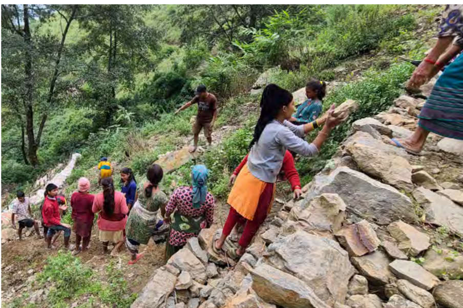
Climate adaptation in action: Following a workshop in Dailekh, Nepal, as part of SNV's WfW Climate Heroes research project , community members work together to create a wall from local materials to protect their water source Credit: SNV / Heman Paneru
