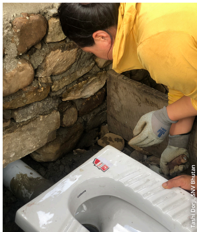
Toilet construction, Bhutan.
