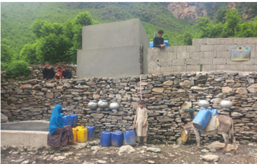
Villagers fill water containers from one of three collection points where a solar-powered pump and system connected to a bore now serve more than 140 households in Yakhdara rural village, Khyber Pakhtunkhwa Province Credit: International Rescue Committee (IRC)/ Anil Kumar
