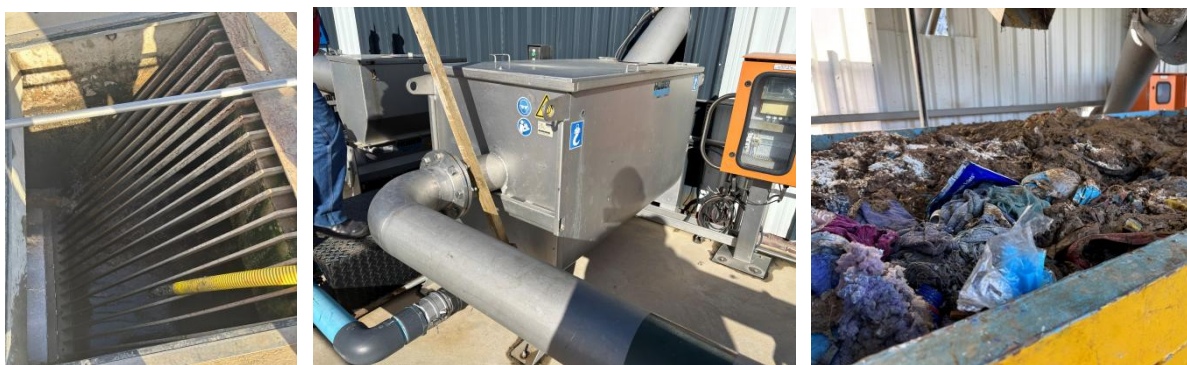
Figure 8: Faecal sludge is discharged into screens and then solid waste is removed before joining the head of works.
