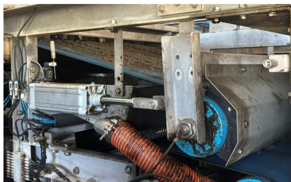
Figure 7: WW sludge belt press at Gwaing WWTW.
