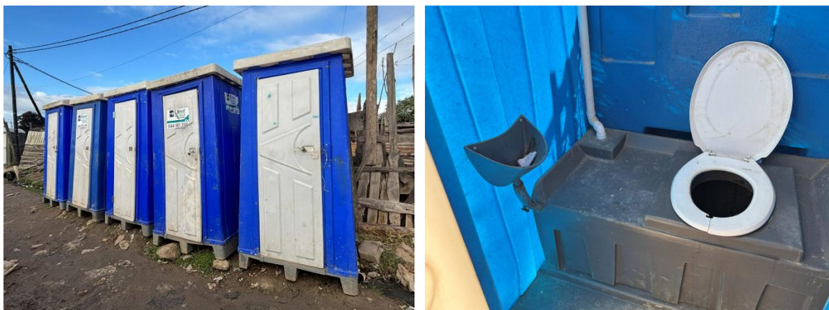
Figure 4: Typical chemical toilets often provided in George LM's informal settlements.
