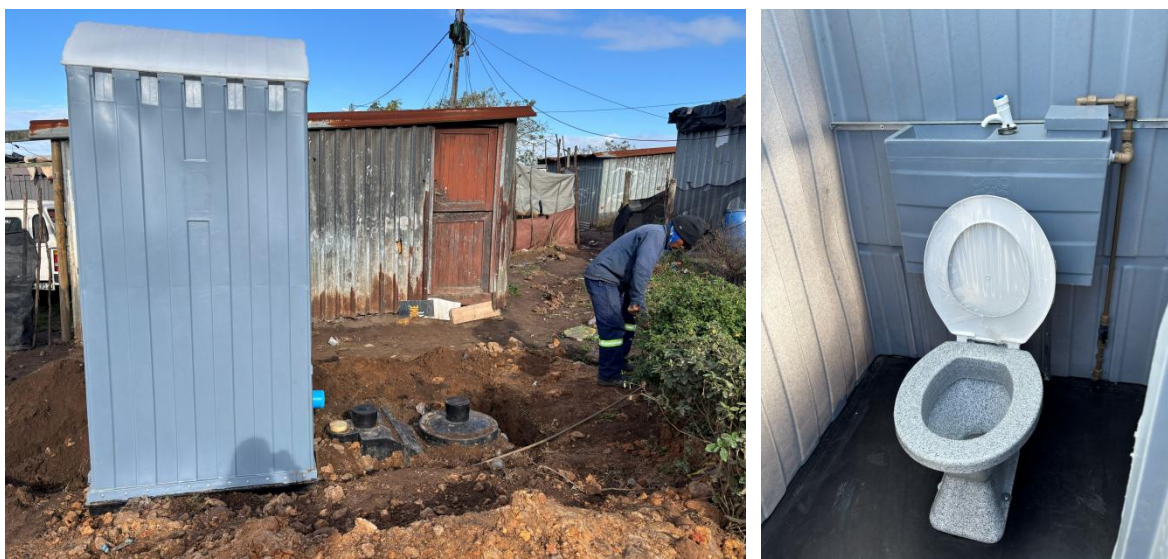
Figure 5: Example of a flush toilet with septic system being installed in one of George LM's informal settlements.
