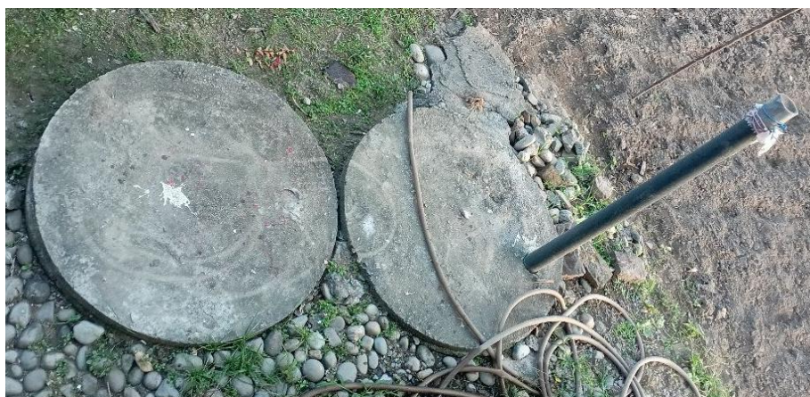
Figure 5: Twin pits installed at the household level.
