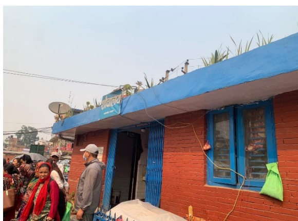
Public toilet at Lagankhel
