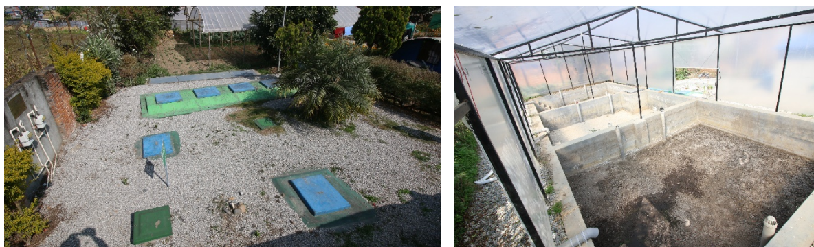
Figure 13: Faecal Sludge Treatment Plant in Mahalaxmi Municipality.
