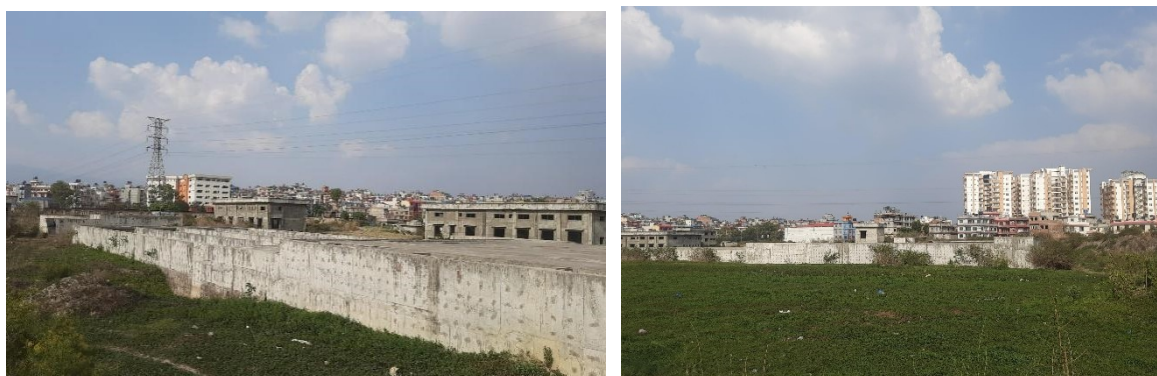
Figure 11: Wastewater treatment plants at Balkumari under construction.
