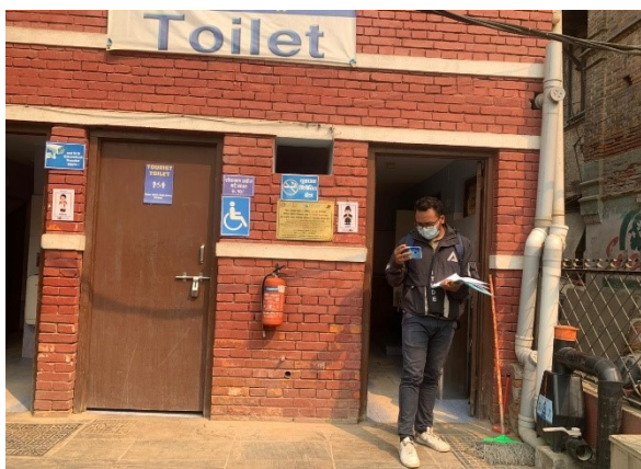
Public toilet at Mangalbazar
