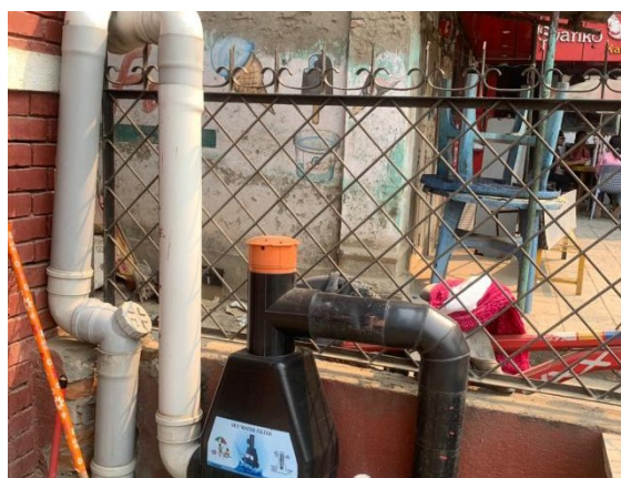
Public toilet at Patan Dhoka
