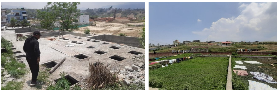
Figure 12: Current status of wastewater treatment plants at ward 28 and 29 of LMC.
