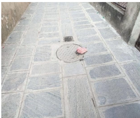
Figure 3: Manhole of the sewer networks connected to households.
