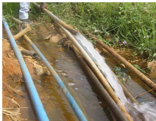
Figure 5.5: Losses due to pipe damage from illegal connections (Krohs, 2004)
