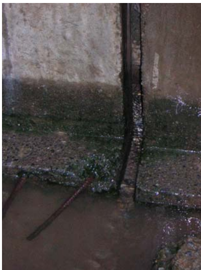
Figure 5. 25: An unprotected water source
