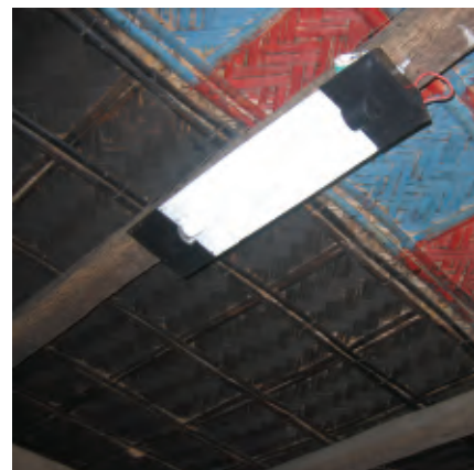
A 85W SHS can support seven 6W tube light like above and a 17" Black and white TV
