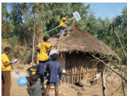
Solar technicians installing a hut
