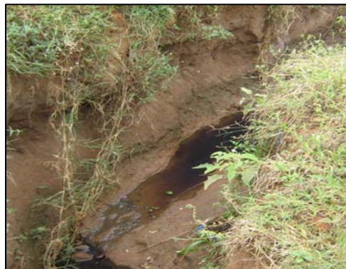
Plate 23: Poor condition of storm drains, Left- Unlined, Right- drain with eminent gully formation. Note the dark brown coloured wastewaters (leachate) carried by the drain.
