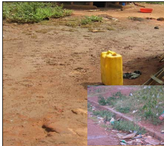
Plate 21: Damp ground following infiltration of stagnant storm water. Typical situation in most low lying areas in KTC, inset is a drain channel that is clogged with solid wastes
