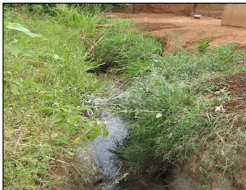
Plate 23: Poor condition of storm drains, Left- Unlined, Right- drain with eminent gully formation. Note the dark brown coloured wastewaters (leachate) carried by the drain.
