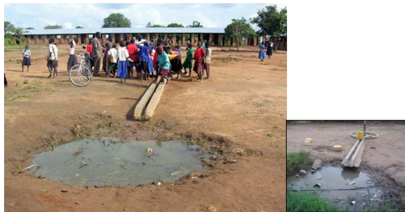
Plate 15: Poor hygiene at some boreholes, the stagnant water can be a potential water source contaminant
