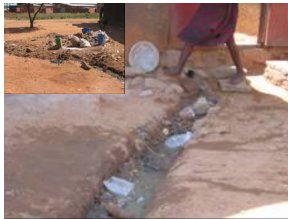
Plate 26: Non sewered grey water in high density areas, Right - bath place with a pipe that leads to the neighbourhoods.
