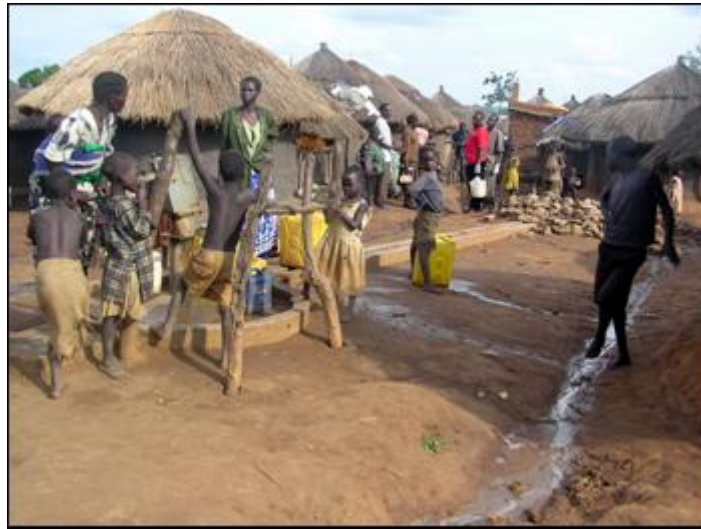
Plate 2: Congested Labujje IDP with unlined storm water and/ or shallow grey water drain adjacent to the borehole
