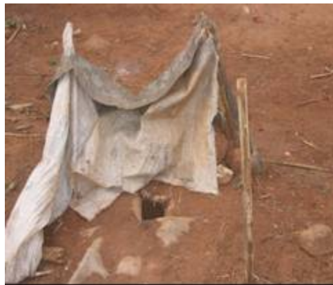
Plate 9: Pit latrine without a super structure
