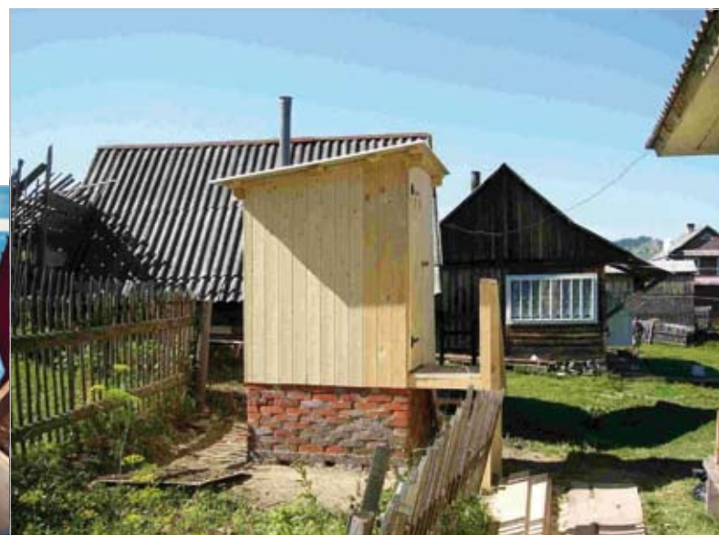
Figure 14: Even for an outdoor setting is a ventilation pipe. relevant Photo by WECF
