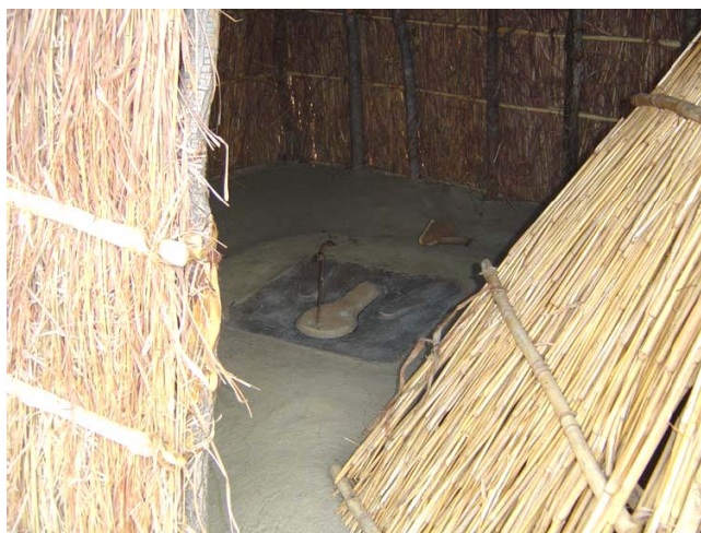
Installed sanplat
