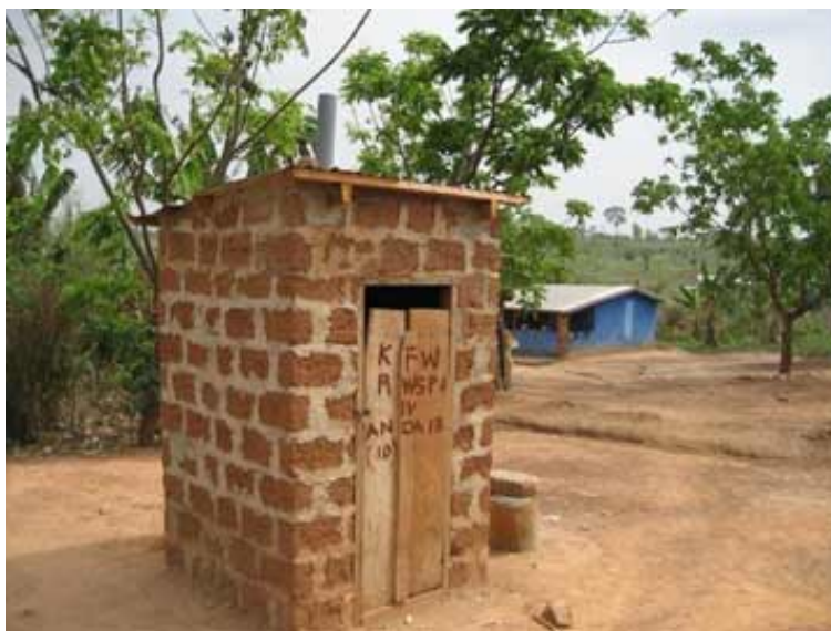
Ventilated improved pit latrine in Ashanti Region
