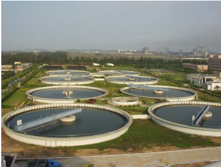
Wastewater treatment plant Haikou
