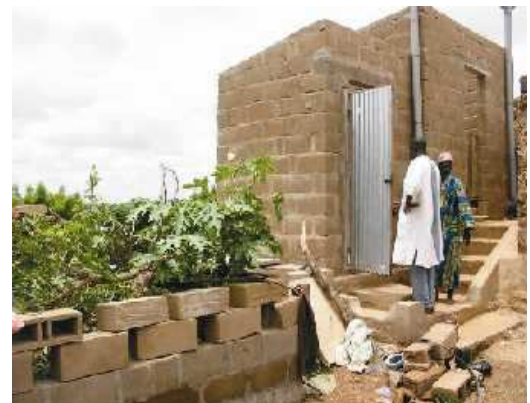
Fig. 3: Ecosan UDD toilet in Koulikoro with shower and greywater garden in 2002 (source: GTZ, 2002).
