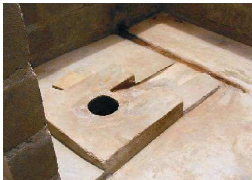
Fig. 6: Latrine urine-diversion squatting pan, where urine drains away to the drainage at the right (source: GTZ, 2002).
