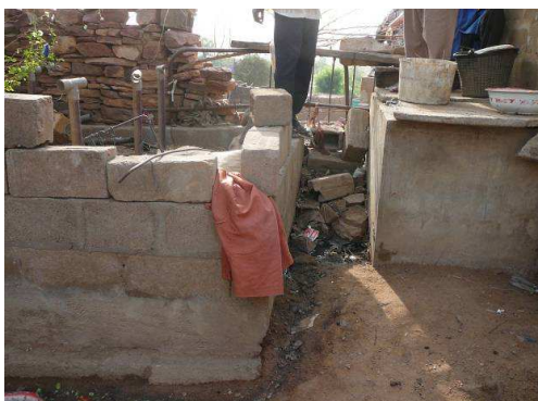
Fig. 4: The same location as Fig. 3: greywater garden on the left side with leaking water from broken pipe (source: Stefan
