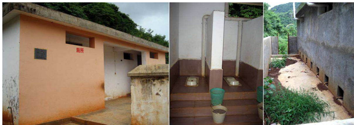
Fig. 3: School sanitation in Yunnan. Middle: Squatting pans. Right: Backside of the building. (Source: P.Feiereisen 2009)
