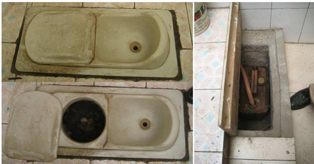
Fig. 1: Left: Squatting pan with movable cover. Right: Urine storage tank integrated into the steps. Example from Shaanxi. (Source: P. Feiereisen 2009)
