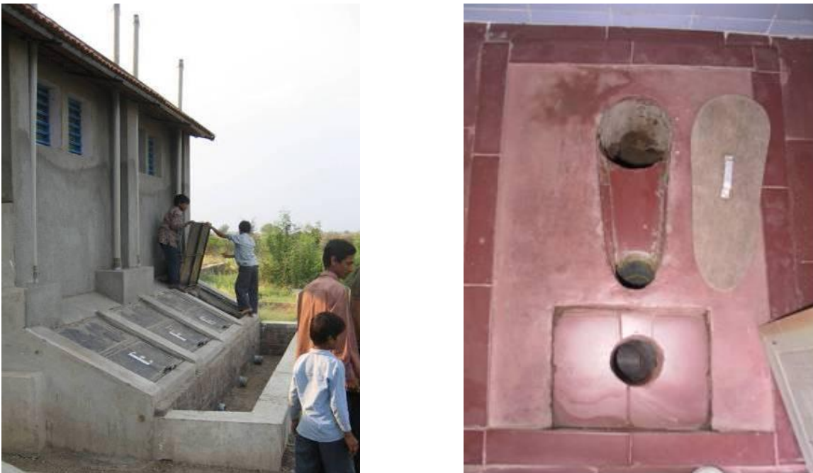
FIGURE 4 UDD toilets at the sanitation facility of the primary school at Rayka village (source: ESF). Left: Faeces dehydration chambers with vent pipes; right: inside view of the toilet: 3-hole UD squatting pan with lowest hole on the photo for anal washing.
