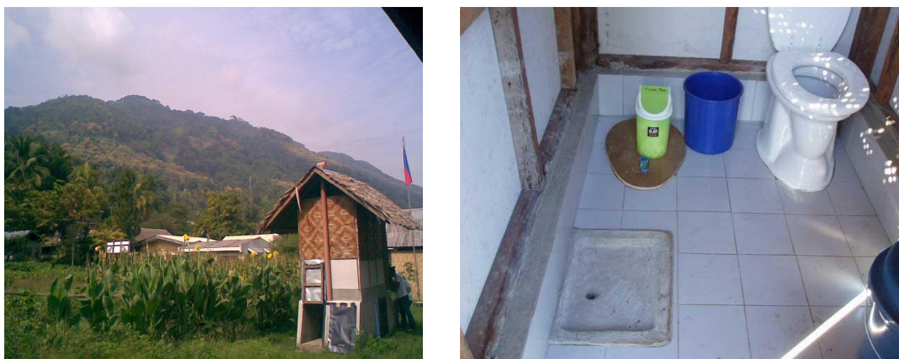
FIGURE 3 Double vault urine-diversion dehydration (UDD) toilet in one of the allotment gardens in Cagayan d'Oro. Left: outside view of toilet; right: inside view of toilet, with anal washing area at the front left (source: R. Holmer and http://puvep.xu.edu.ph/ecosan_toilet.htm )
