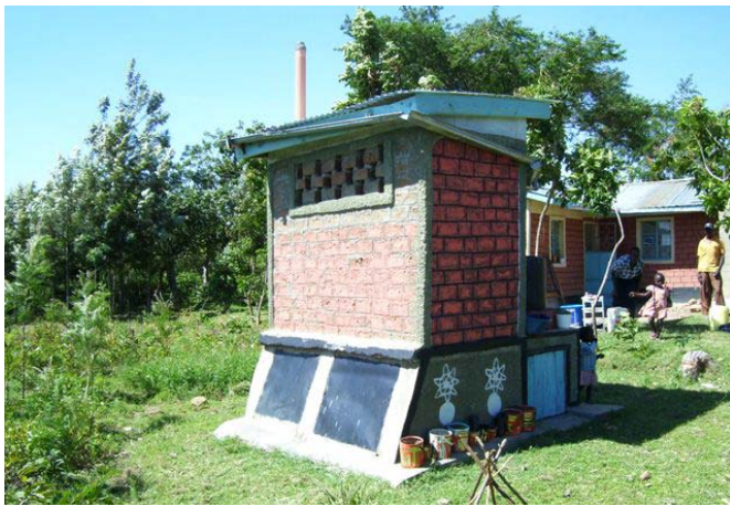
Fig. 6: Back view of household UDDT near Bungoma town in Western Province with two faeces vaults and ventilation pipe (source: Moses Wakala, GTZ-Kenya, Jan. 2010). Note: The inclination of faeces vault doors is not necessary for proper function – see Section 11. Moreover note the toilet is in relative close distance to house.
