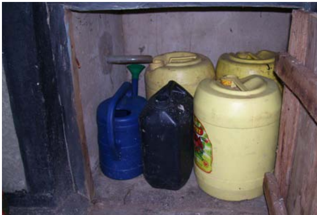
Fig. 11: Inside of urine storage vault with a number of urine containers (Source: Moses Wakala, GTZ-Kenya, Jan. 2010).
