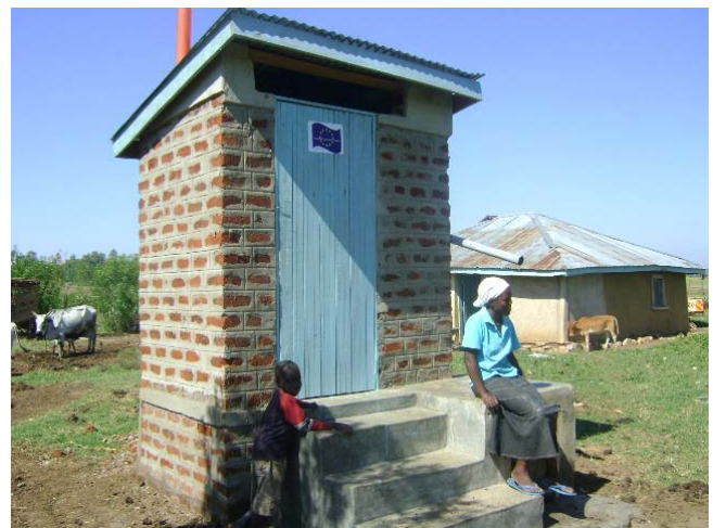
Fig. 3: Rural household UDDT in Nyanza Province (source: Paul Mboya, GTZ-Kenya, Aug. 2009 – Note distance between house and toilet is approx. 20 meters)
