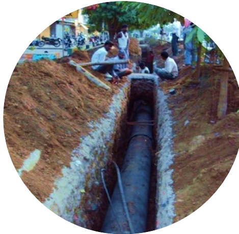
Sewerage network maintenance
