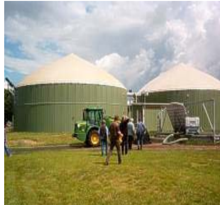
Decentralised biogas plant
